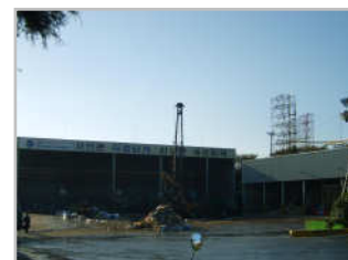
• Wastewater Treatment and Storage Facility
