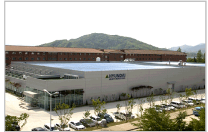
· Eumseong Solar cell-producing Plant
