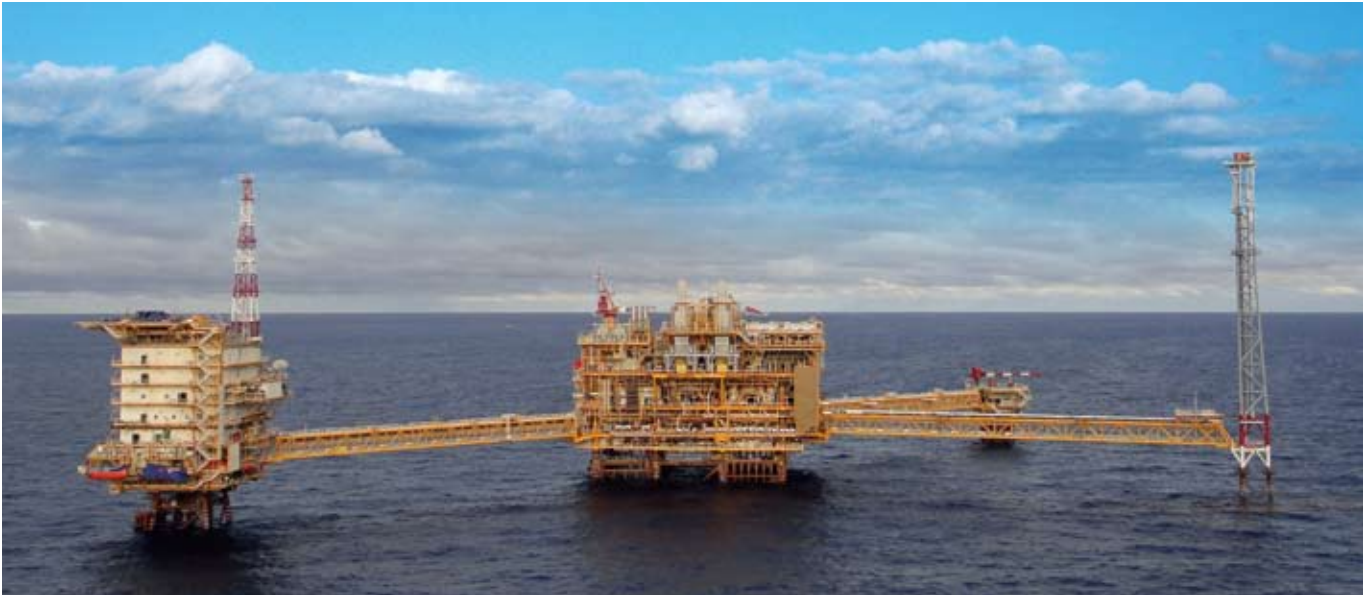
Bongkot South platform installation In August 2011, we installed this 30,000-ton processing platform for PTT Exploration and Production of Thailand. Designed to process 385 million square cubic feet of natural gas and 15,000 barrels of condensate per day, the platform is now operating in the Great Bongkot South field, 600 km southeast of Bangkok.
