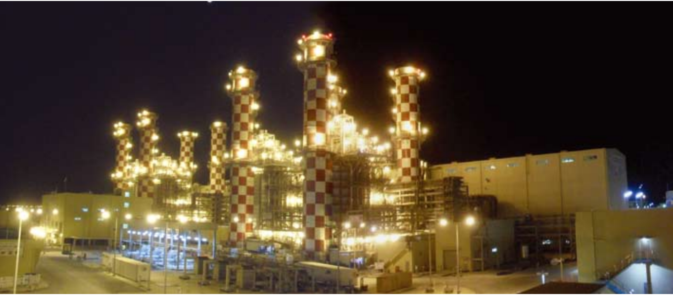
Al Dur IWPP completion Ordered in 2008 by the Al Dur Power and Water Company, this USD 1.7 billion EPC build-own-operate project began commercial operations in early 2012. The 1,245 MW combined-cycle power plant produces the equivalent of almost one-third of Bahrain's total existing generation capacity, while the adjacent reverse osmosis desalination plant delivers 48 MIGD of water to meet the kingdom's growing needs.
